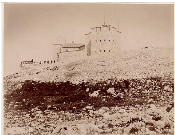
Sl. 3.1. – Tvrđava Kličanj (Werk I) Fig. 3.1 – Kličanj Fortress (Werk I)
